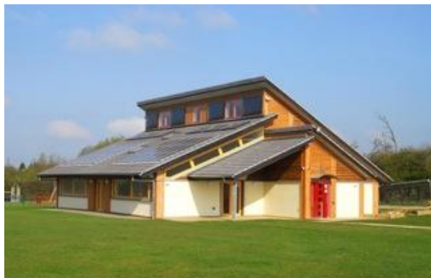
[Solar Panels on community hall at OHMG]
